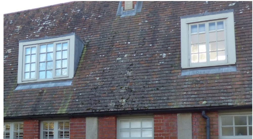
Figure 24: Two sets of casement windows on a building within the Conservation Area. The one on the right has even sightlines.
