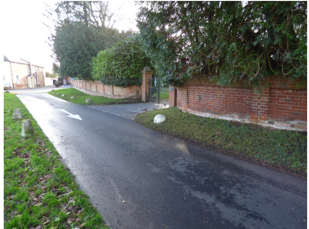
Figure 52: The brick wall to Crown House makes an important contribution to the Conservation Area.
