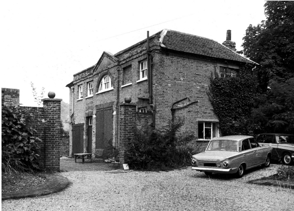
Figure 6: The Coach House to The Old House is a subservient building to the main house but is of a high architectural character. 8
