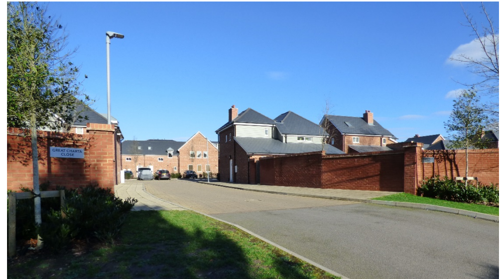
Figure 56: The high density of development of Great Charta Close urbanises the setting of the Conservation Area.
