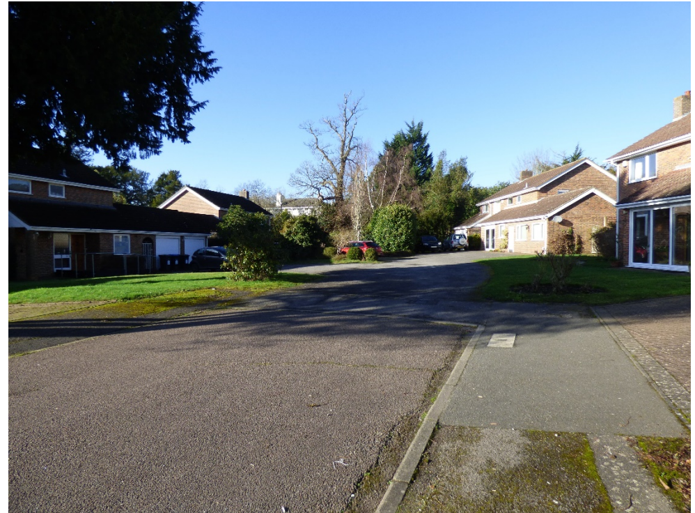
Figure 61: The houses in Oak Tree Drive and Bulkeley Close do not reflect the character and appearance of the Conservation Area.
