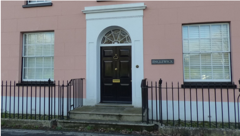
Figure 25: An example of a classically inspired porch with a six panel door and eighteenth century style fanlight.
