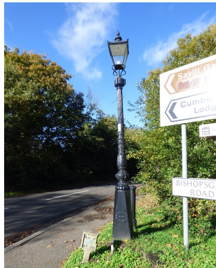
Figure 43: The cast iron lamppost in Englefield Green is one of the four locally listed heritage assets in the Conservation Area.
