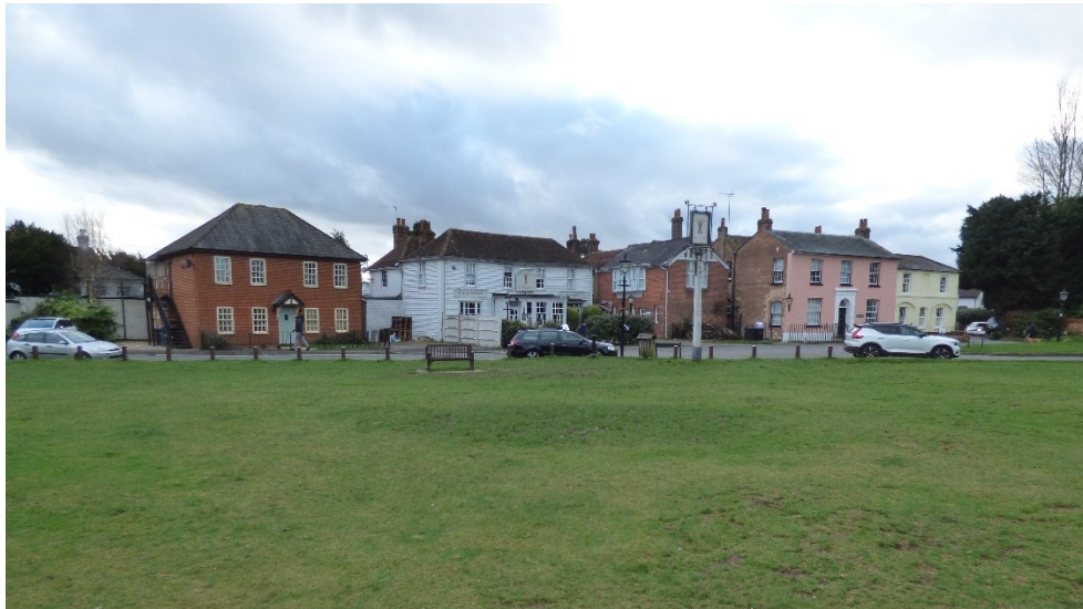
Figure 18: The buildings along Barley Mow Road are set hard against the pavement in contrast to many of the villas.
